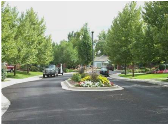
Median islands serve to reduce the travel way on local streets and add aesthetic qualities.
