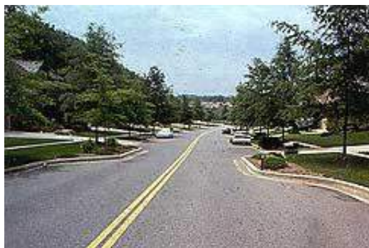
Chicanes are effective ways to physically narrow the roadway and slow vehicle speeds.
