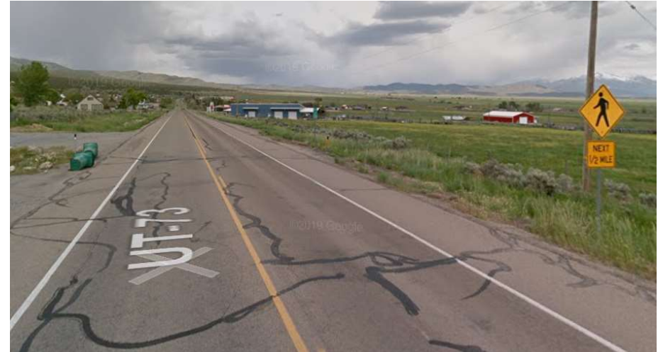
Portion of SR-73 near Cedar Fort, Google Maps, 2022.
