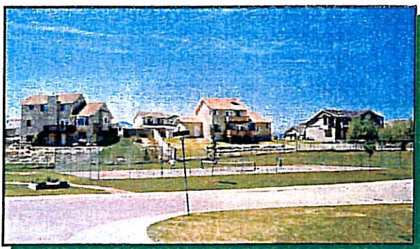
Figure 4-4: Contaminated soil used as backfill material under a road and a tennis court.
