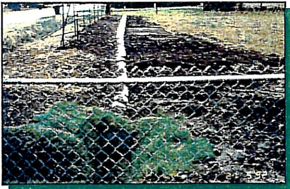
Figure 4-14: Pipeline replacing contaminated ditch.
