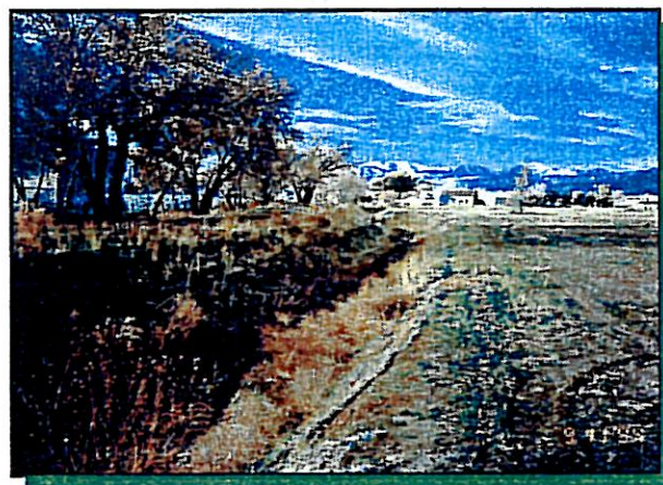
Figure 4-11: Photo of the contaminated ditch adjacent to a residential neighborhood, prior to cleanup.
