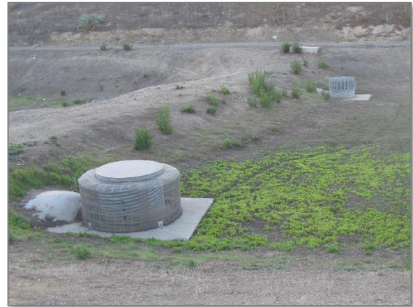
Figure 4: Multi-stage overflow outlet with trash screen
