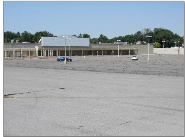
Figure 1: Impervious parking lot with no pervious areas or storm water quality features
