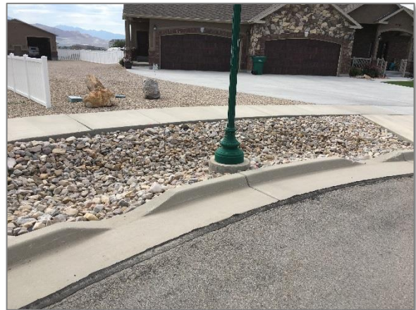
Figure 8: Curb cuts to a rock lined swale.
