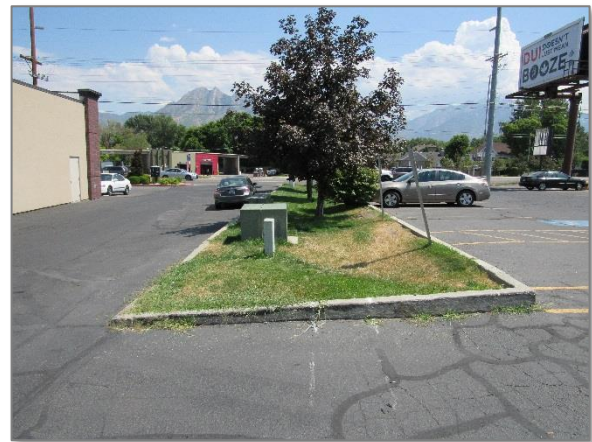
Figure 2: Potential curb cut location that could be retrofitted into a swale
