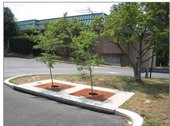
Figure 13: Proprietary tree box filter
