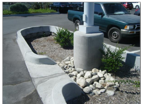
Figure 3: Retrofitted island curb within parking lot
